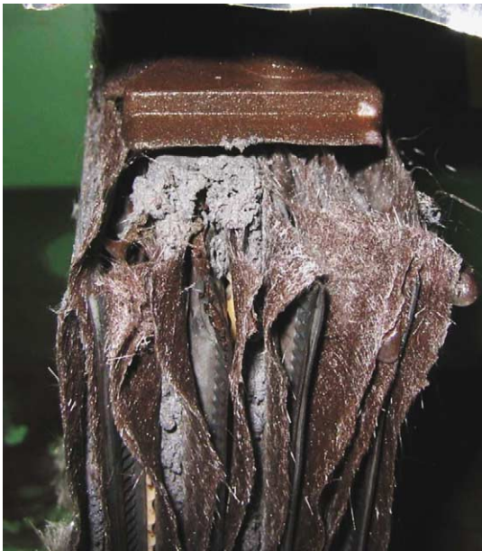
Fig. 4. Photograph of short-circuit at the top of the electrode stack in a compressed application.
